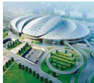
Beijing South Railway Station
