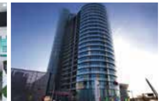
Tianjing Electric Power Company
