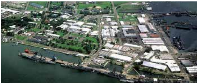
Subic Bay solar power station in the Philippines
